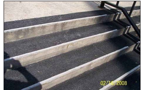
The steps 5 years later, still in excellent condition.
